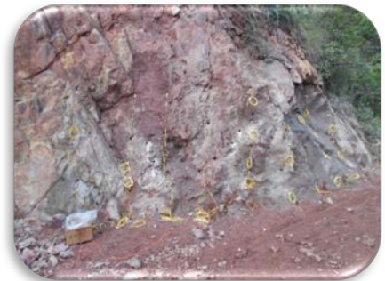
Figure 1 - Detonator cord ready for 1 st blast initiating Portal construction.
